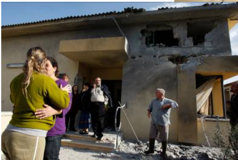
Family in front of its ruined house in the village of Tequma, not far from the city of Netivot (Gil Cohen Magen for Reuters, December 24).
